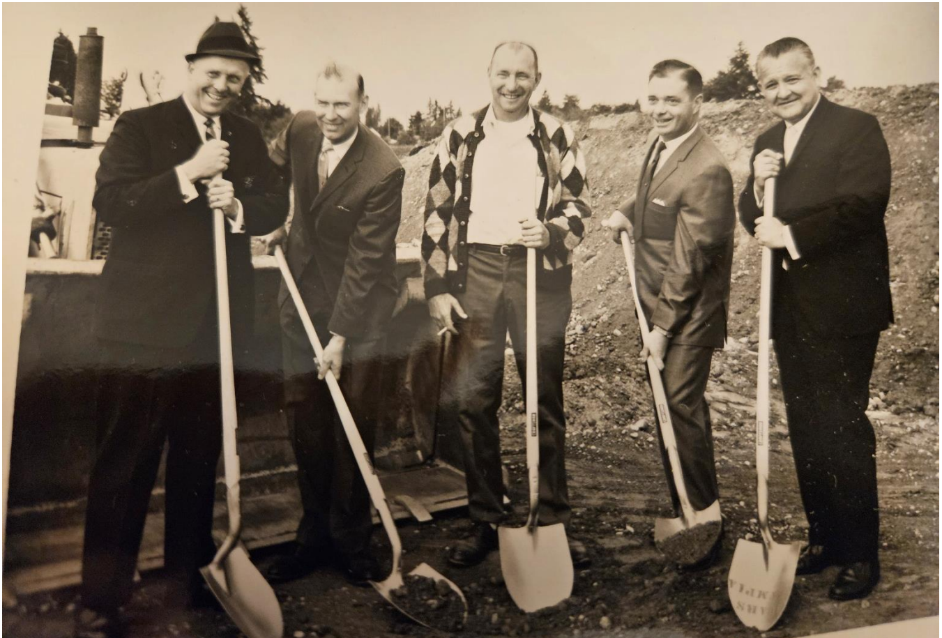
Groundbreaking for the Sears store at South Sound Center. Bob Blume is second from the right.
